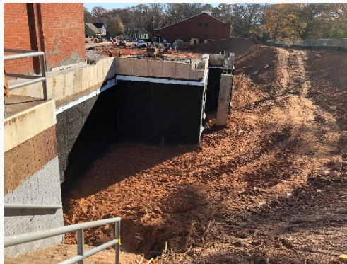
Waterproofing & Backfill
