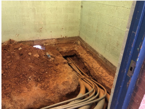
MEP OH rough, Electrical feeds, new slab edge formwork
