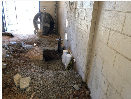
MEP under slab rough, new water stub up retaining wall backfill
