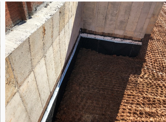
MEP under slab rough, new water stub up retaining wall backfill
